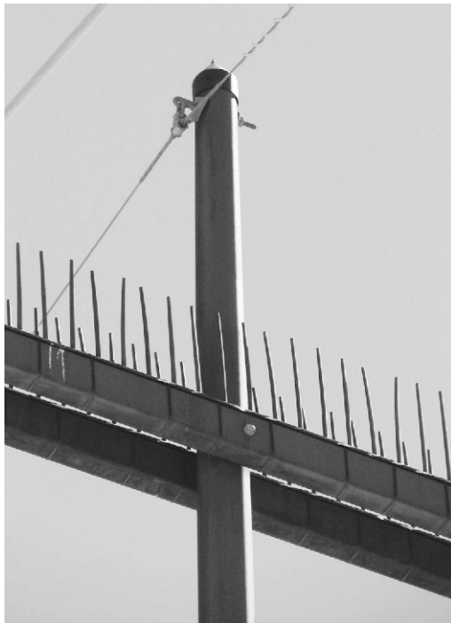
Figure 1. Raptor perch-deterrent devices (Zena, Inc., Odenville, AL) used on cross-arms and pole-tops of H-frame power-line support structures in southwest Wyoming, USA, in 2007.
