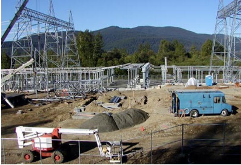
FIGURE 1.7-9 Substation under Construction (Source: BPA)
