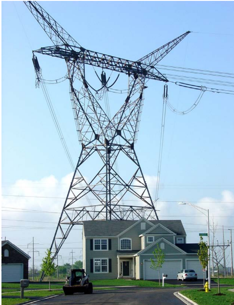
FIGURE 1.6-3 Deviation Tower in a Residential Neighborhood (Source: Argonne Staff Photo)
