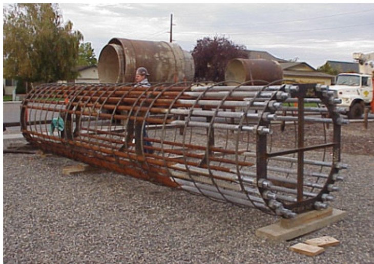
FIGURE 1.7-4 Anchor Bolt Cage and Reinforcing for Tower Foundation Construction (Source: BPA)
