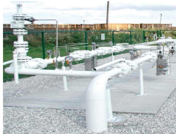
FIGURE 3.9-8 Typical Natural Gas City Gate
