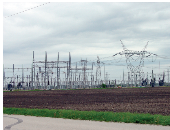
FIGURE 3.9-4 Transmission Lines Leaving Substation
