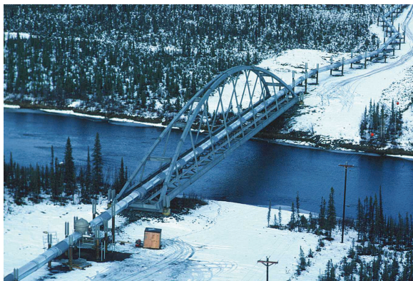
FIGURE 3.9-9 Trans-Alaska Pipeline Bridge over Gulkana River
