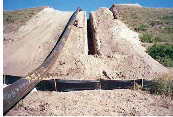
FIGURE 3.9-2 Trenching in Preparation for Installation of Gas Pipeline
