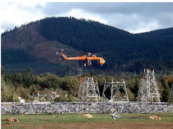
FIGURE 3.9-1 Towers under Construction
