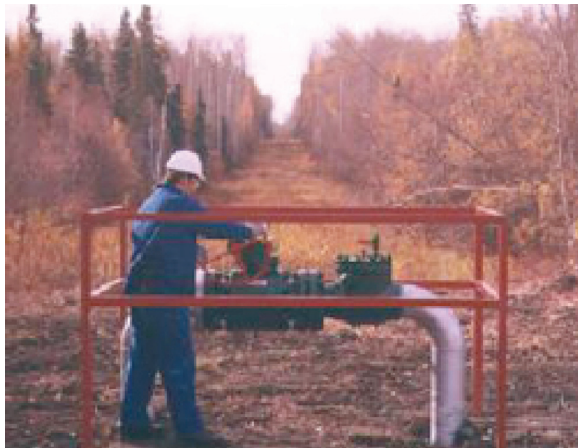
FIGURE 3.9-5 Natural Gas Control Valve
