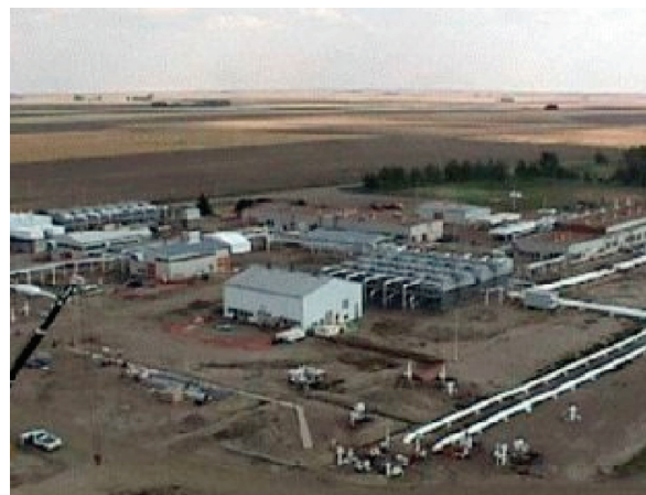
FIGURE 3.9-6 Typical Natural Gas Compressor Station
