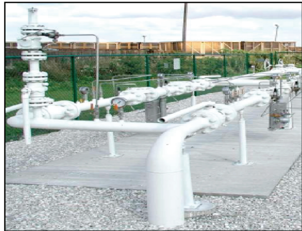
Typical natural gas city gate
