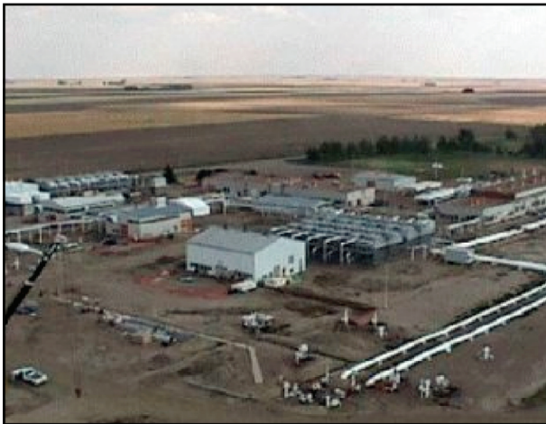
Typical natural gas compressor station
